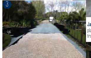
**JakMat** *Geocell* contains the materials in place, for heavy duty vehicles such as water trucks.
